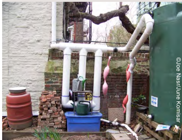
New York, USA. Rainwater collection system installed by GrowNYC in a community garden
